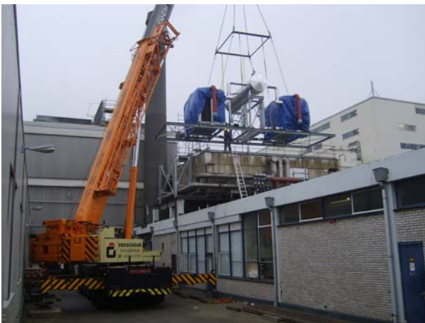
The new ice water installation is based on the "falling film" principle.
